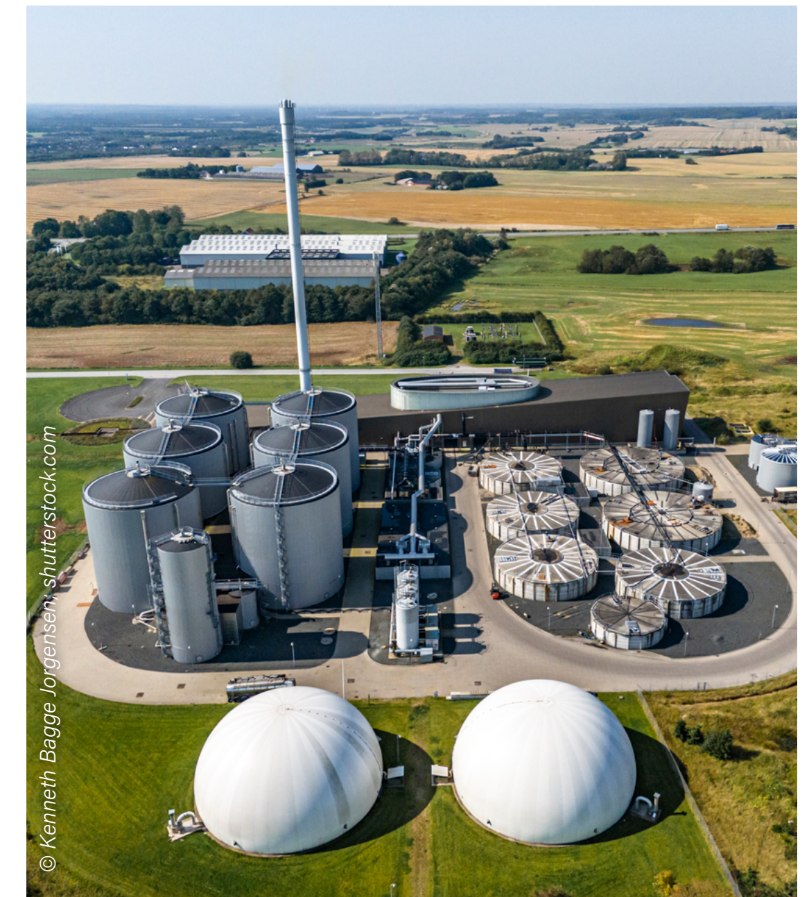
Biogas production, Holstebro, Denmark
